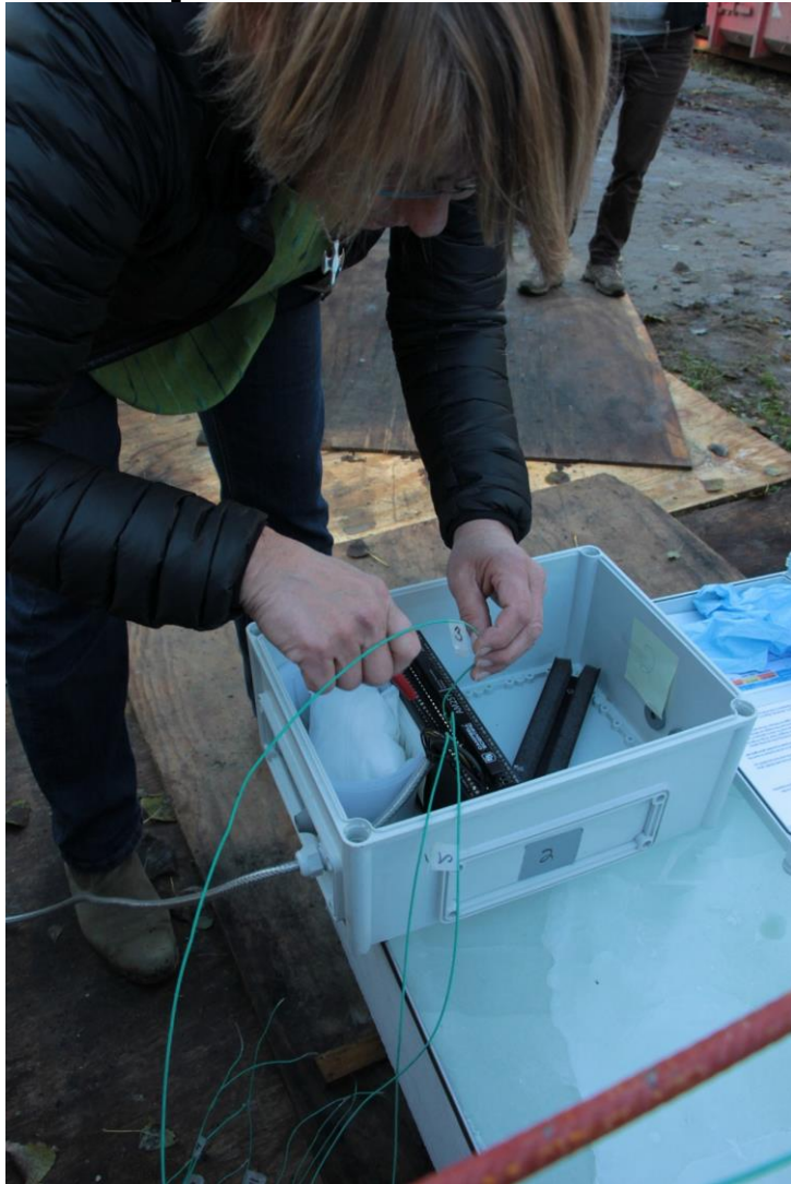
Connection of 20+ temperature sensors
